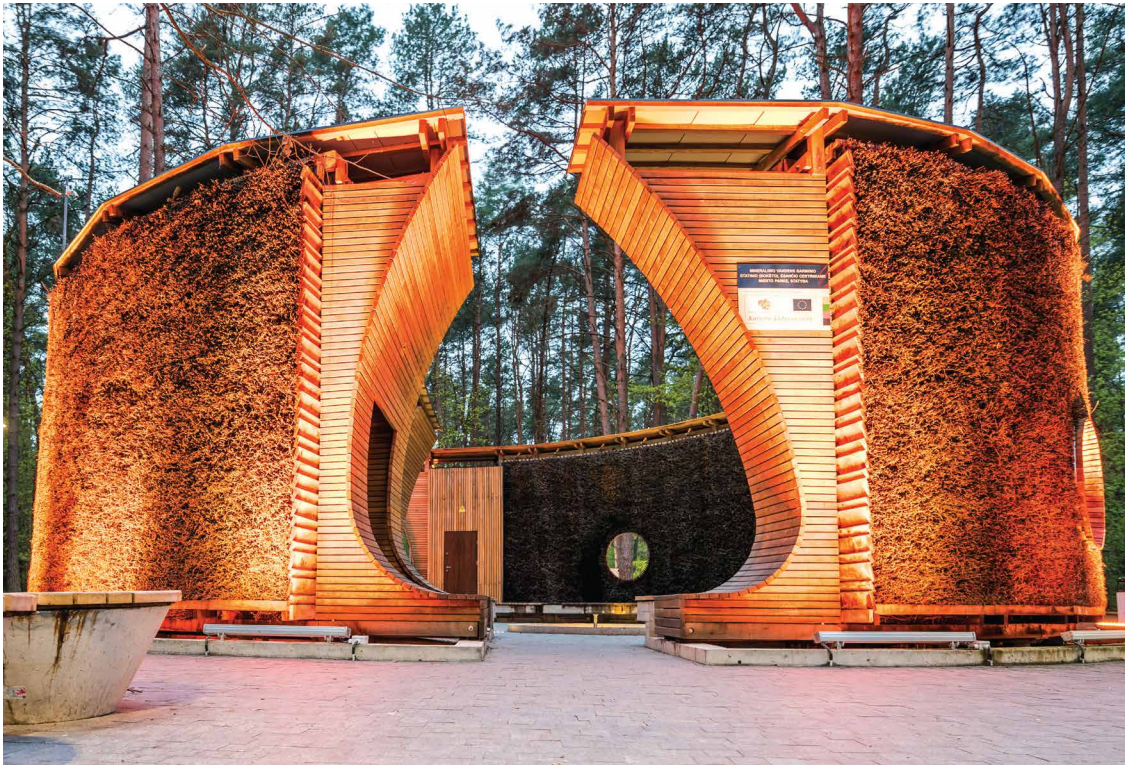
Birštonas Mineral Water Evaporation Tower
